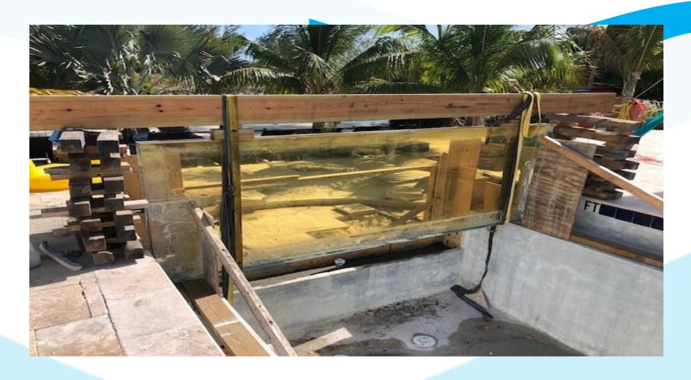
**Choosing The Right Acrylic:** SPW provides UV inhibited, pure methyl methacrylate acrylic panels. Non-UV Inhibited acrylic will inevitably turn from clear to yellow in a matter of months.
